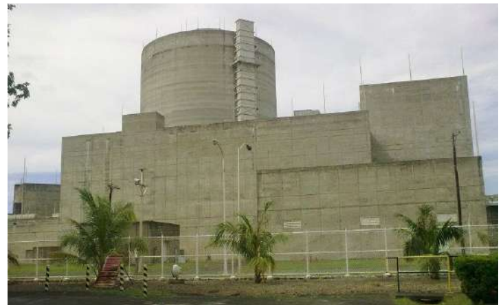
The Bataan Nuclear Power Plant in the Philippines, built with 'petrodollar loans' to the Marcos regime, was completed but never launched.
